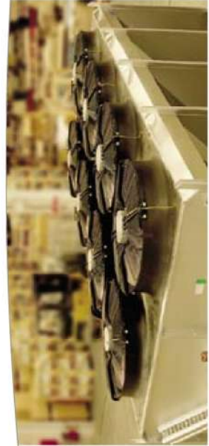
Meticulous control of fans saves energy and keeps noise and draft at a minimum.
